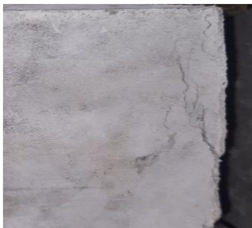
Fig. 10. Cracking in the sample with 0.4% fibers.
