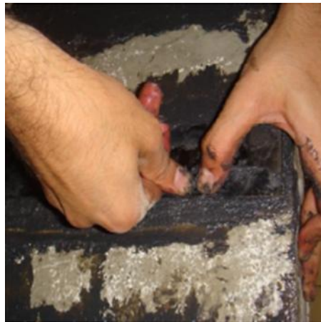
Fig. 8. Installation of FRP fibers on resin.
