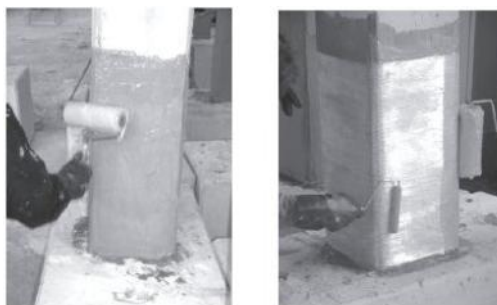
Fig. 5. Wet gluing method [13].
