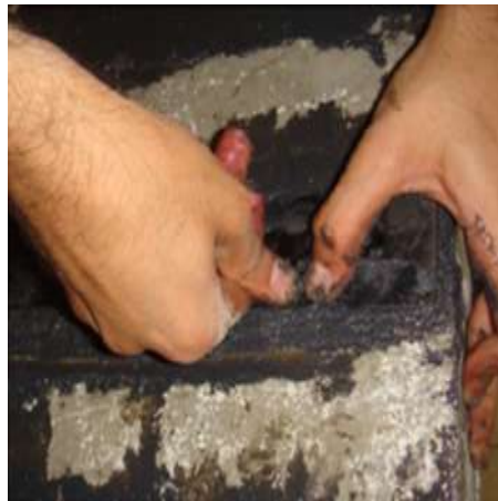
Fig. 8. Installation of FRP fibers on resin.
