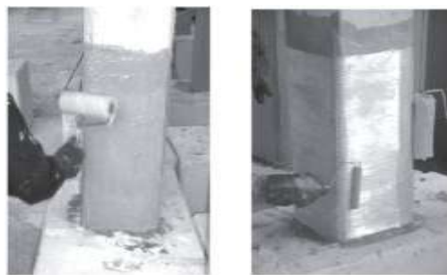
Fig. 5. Wet gluing method [13].
