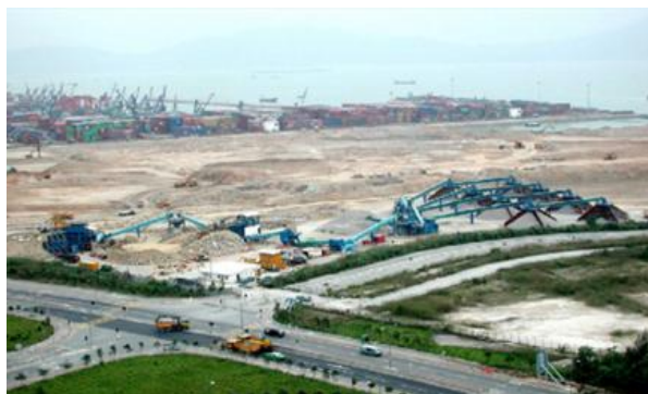
Fig. 1. A picture of a concrete recycling center in Hong Kong.
