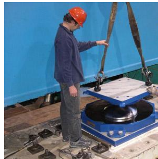
Fig. 4. Installation of pendulum separators.
