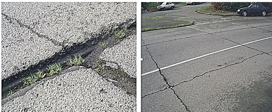
Fig. 8. Reflective cracking [61].
