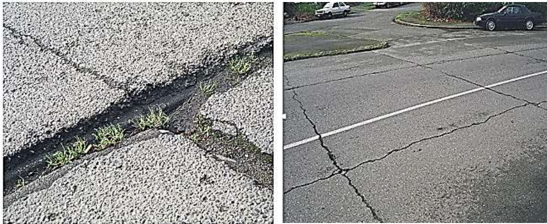
Fig. 8. Reflective cracking [61].
